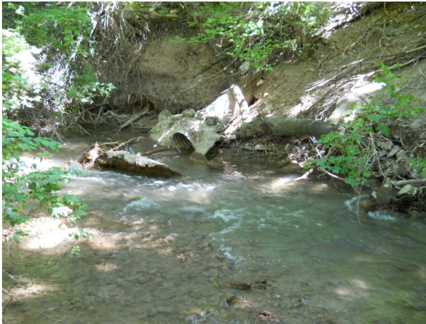
Photo 24: Emigration Creek above 2100 E, looking upstream
